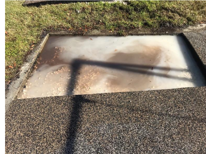
Cut surface at playground for Irrigation repair
